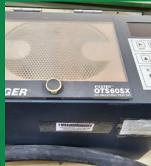
Transformer oil testing
